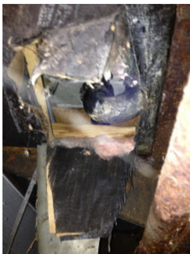
Leak at bathroom trap under mobile home
