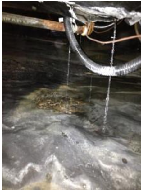
Leaking Plumbing System under a Mobile Home Laundry Area
