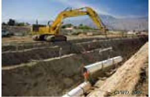
Installation of 54-inch Mid-Valley Pipeline for delivering recycled water
